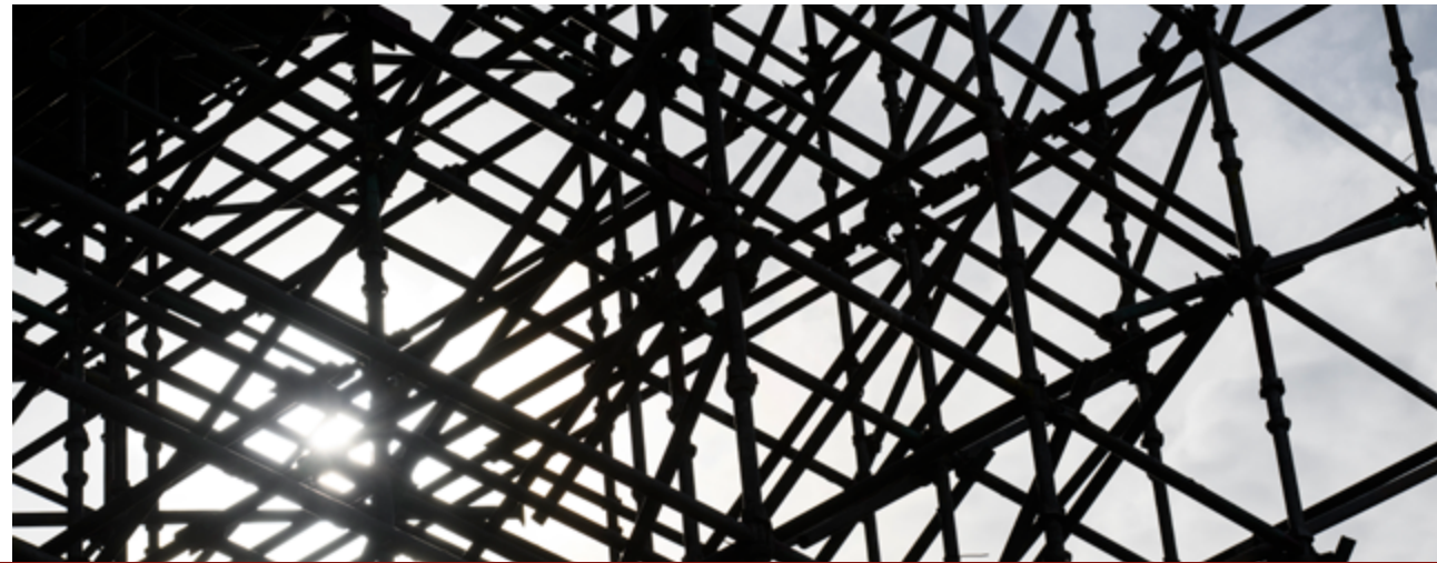
Glasgow Harbour | Vinci Construction
